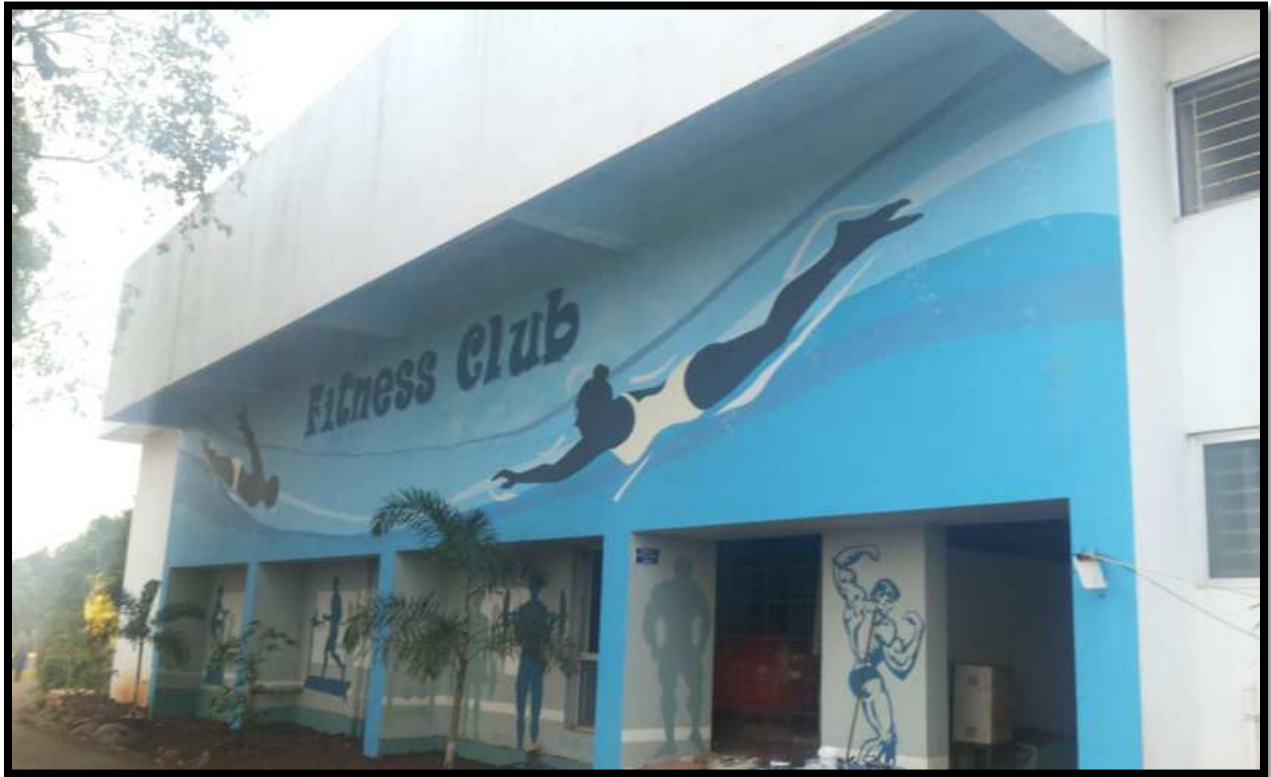
FITNESS CLUB (GYMNASIUM AND SWIMMING POOL BUILDING)
